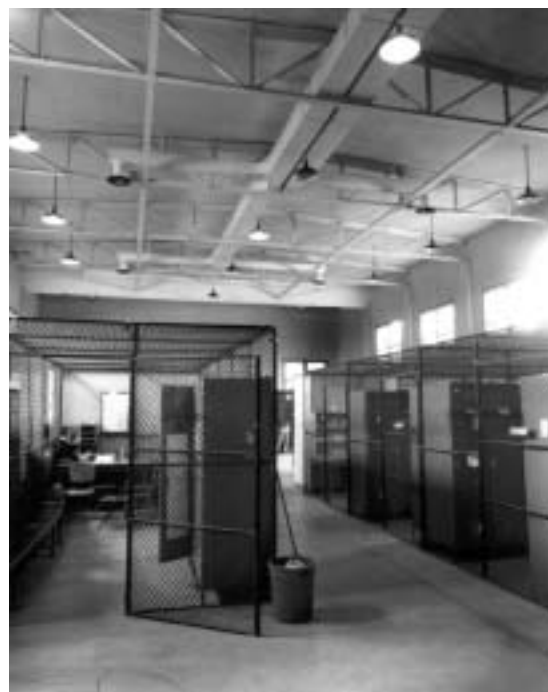
RECREATION ROOM, LOOKING SOUTH. WIRE CAGES WERE CONTEMPORARY ADDITIONS FOR STORAGE AND OFFICE SPACE. PHOTOGRAPH BY TERRY RISHEL (SEPTEMBER 2002).
